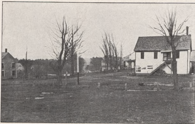
Looking West from Madison Corner.
